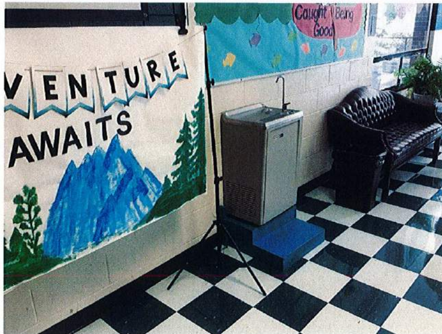
Pinnacle Figure 4: Non-ADA compliant water cooler
