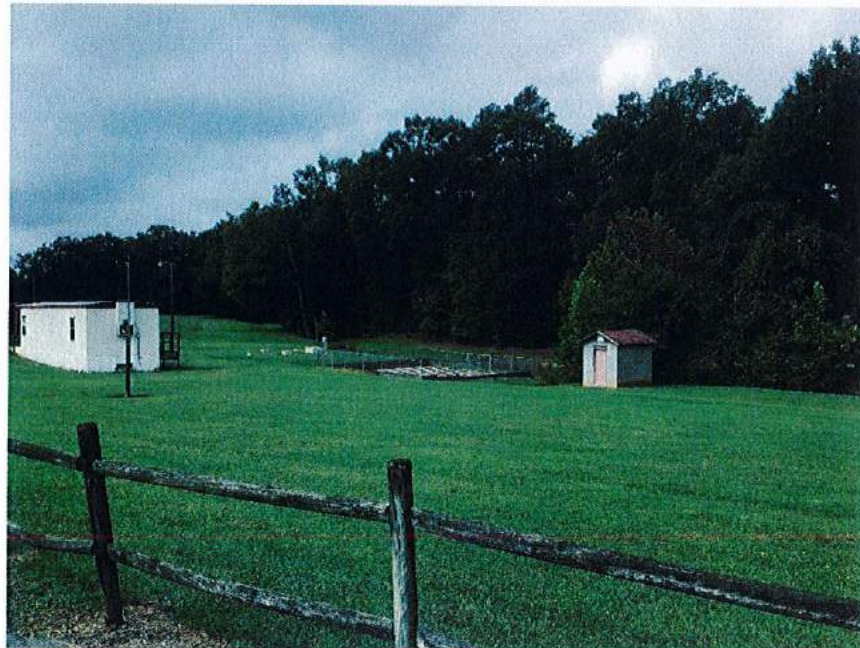
Pine Hall Figure 2: Sand filter bed
