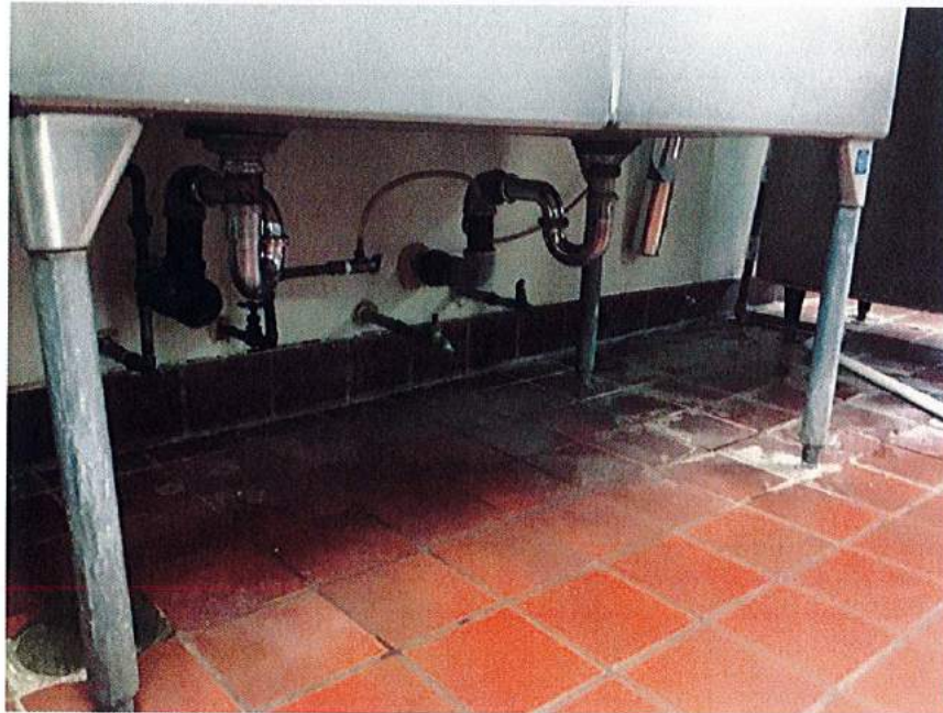
Lawsonville Figure 2: Direct connected 2 comp sink
