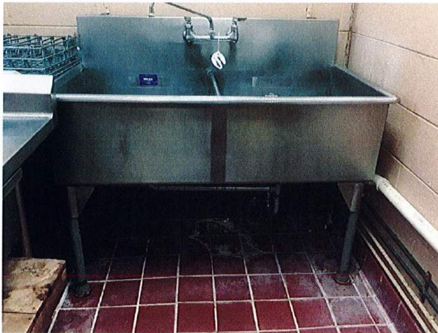
Pine Hall Figure 4: Direct connected sinks
