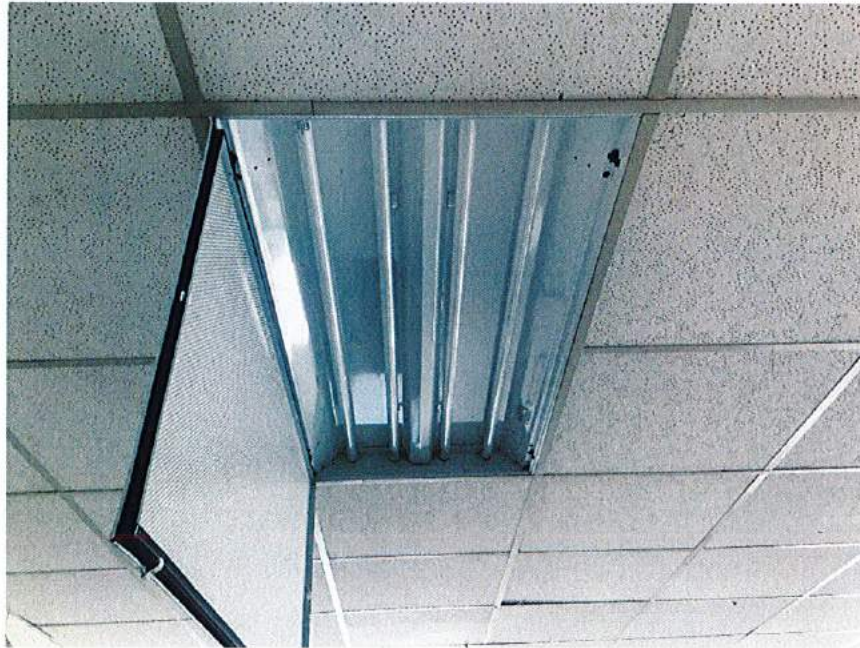
Pinnacle Figure 14: T-8 Lights
