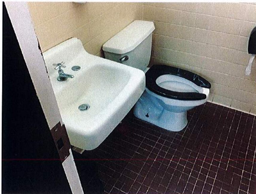
Pinnacle Figure 2: Tank type water closet
