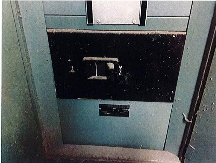
Pinnacle Figure 11: Separate building gym. FPE Main
