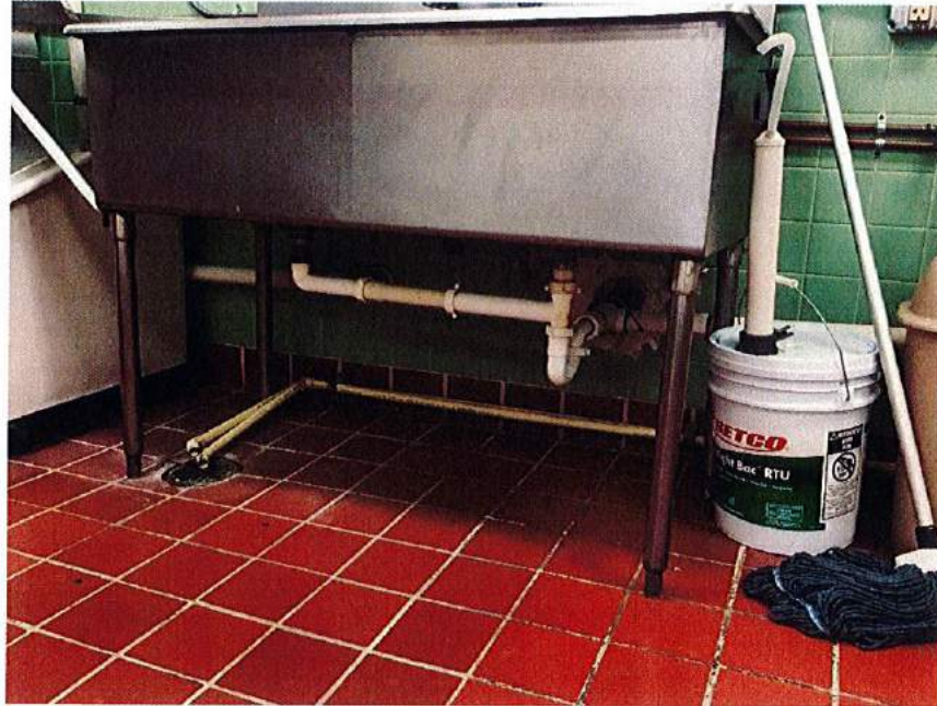
Pinnacle Figure 1: Direct connected sinks
