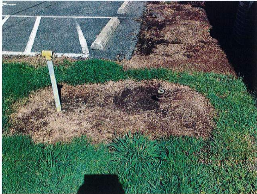
Pinnacle Figure 6: Underground fuel oil tank
